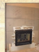
Wire Mesh applied over drywall.
