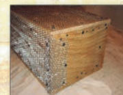
Scratch-coat of mortar applied.
