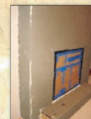
Scratch-coat of mortar applied.
